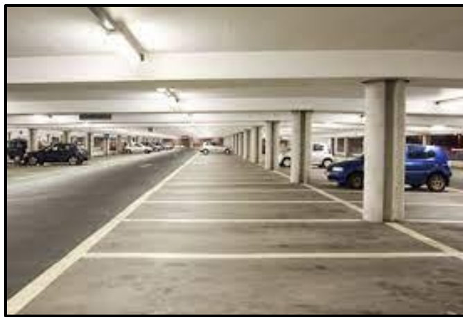
Figure 5. Visual representation of entirely concrete infrastructure of building (courtesy of concretoparking.org)
