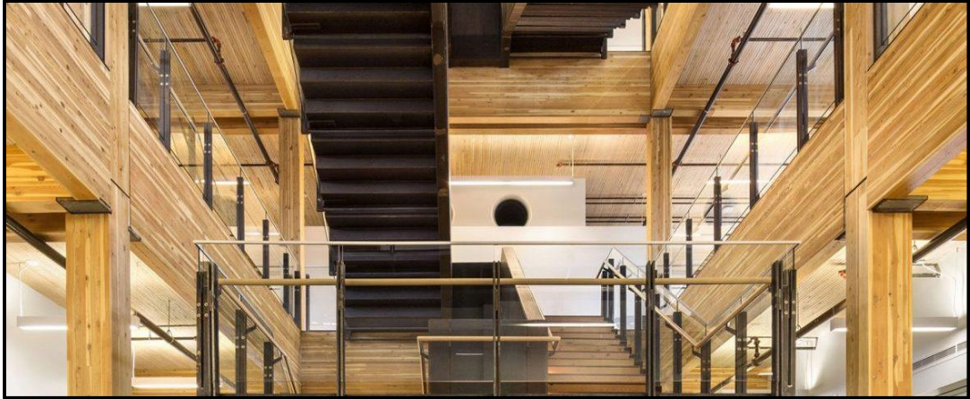
Figure 3. Visual representation of an integrated steel and mass timber design (courtesy of pesengineers.com)
