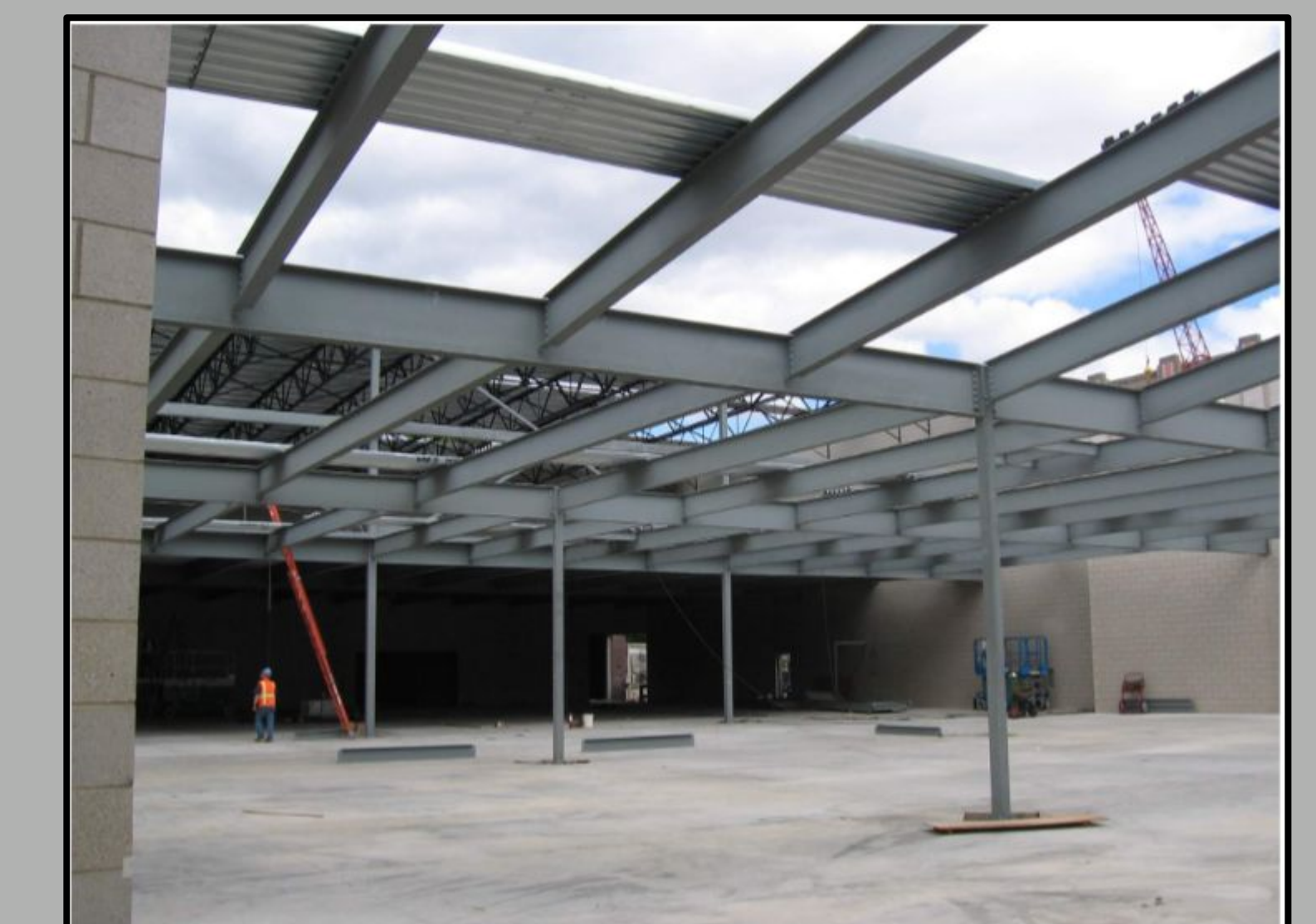
Structural steel members during construction (OSU Basketball Center Working- Presentation)
