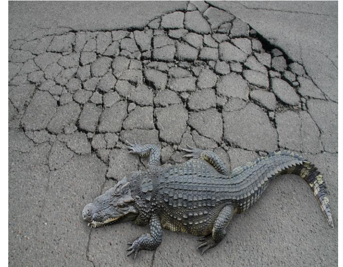
Fatigue cracking
