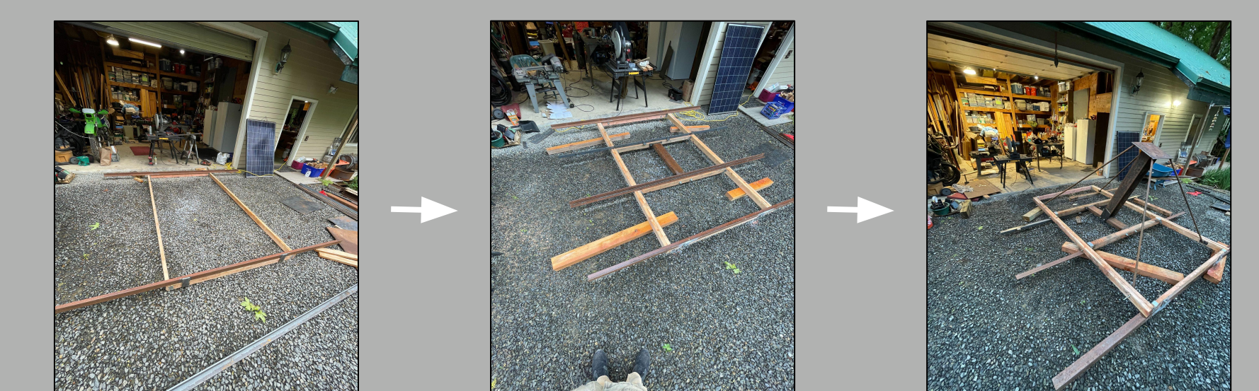
Figure 7: The building process of the upper frame.
