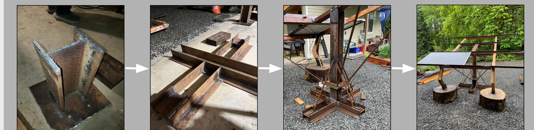
Figure 8: The building process of the base.
