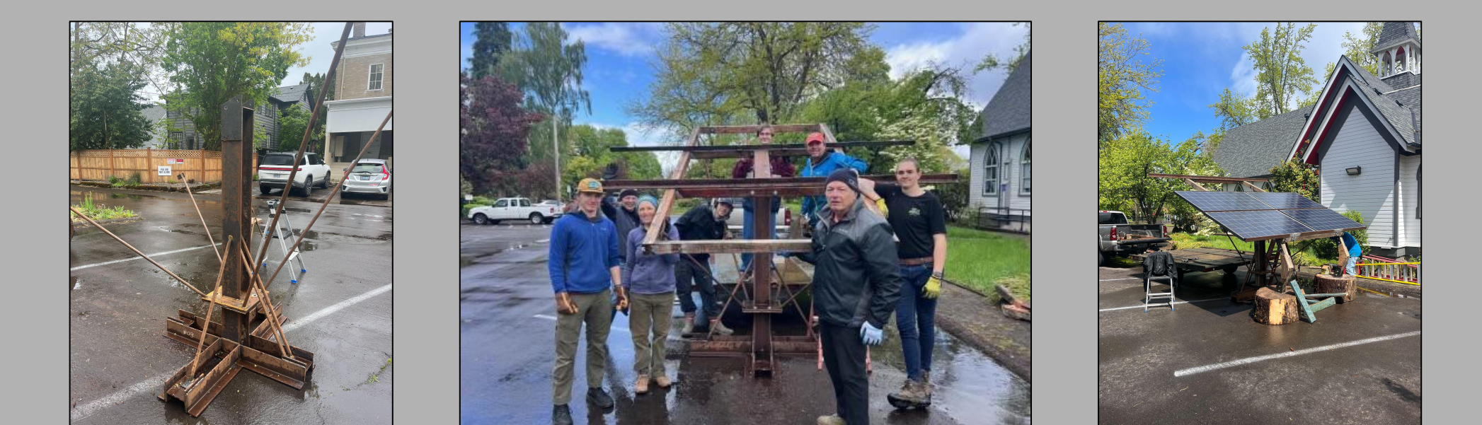
Figure 9: Installation of Oculus
