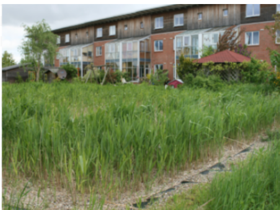
Figure 3: Subsurface flow wetland
