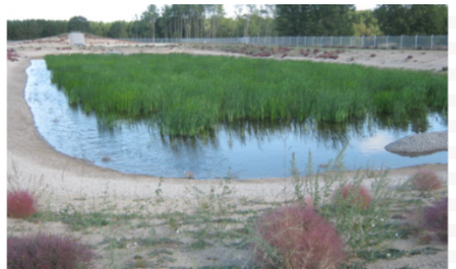
Figure 2: Surface Flow Wetland (Leachate Management Specialists)
