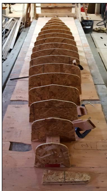
Aligning Cross Sectional Ribs
