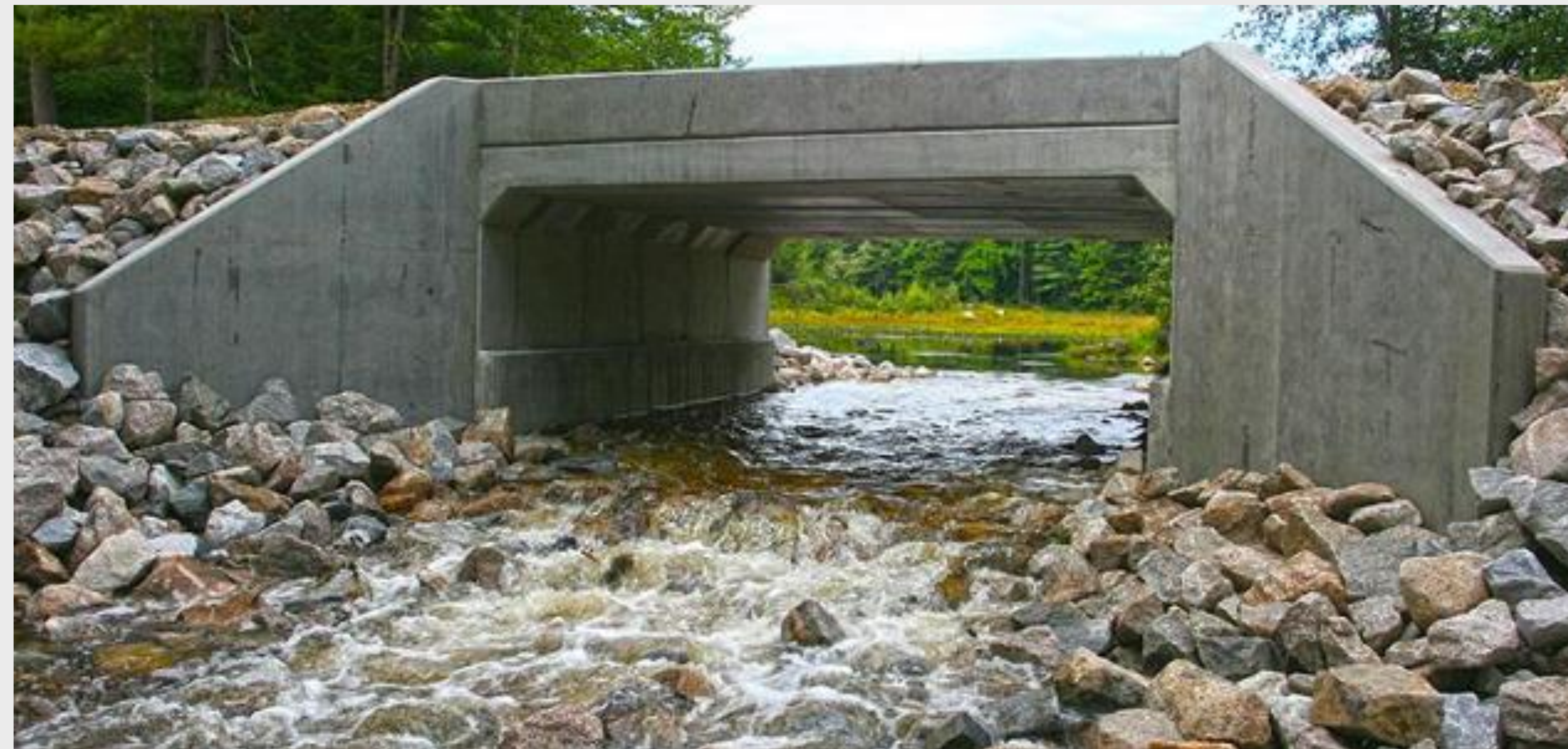
Final Slab Culvert Design
