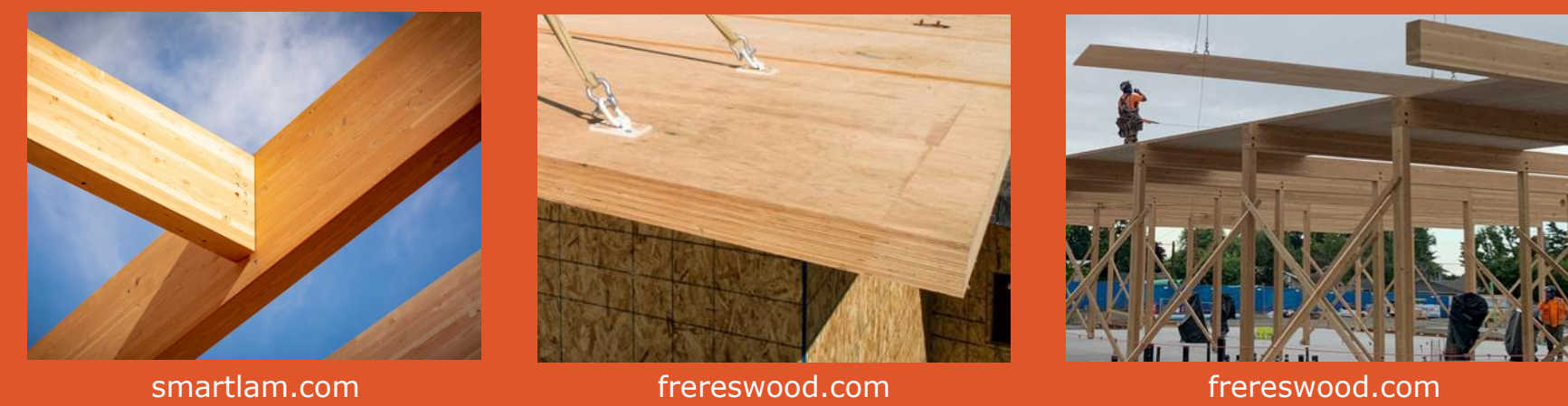
Left to right: Glulam beam to girder connection, example of MPP use, and example of glulam beam and column gravity load system
