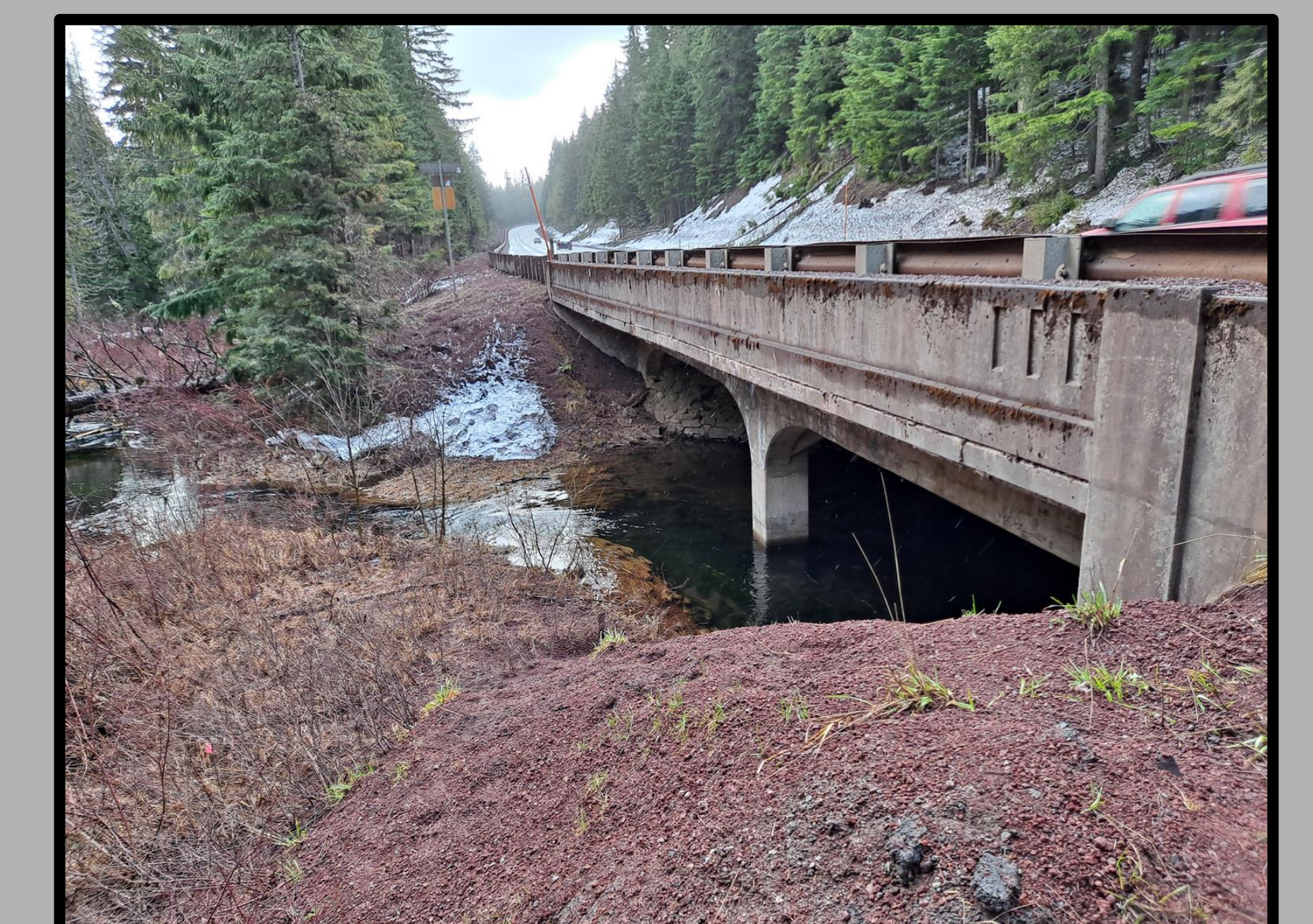
Existing Bridge and Creek
